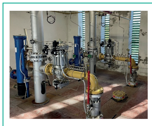
Figure 7 Methane gas distribution PRMS
