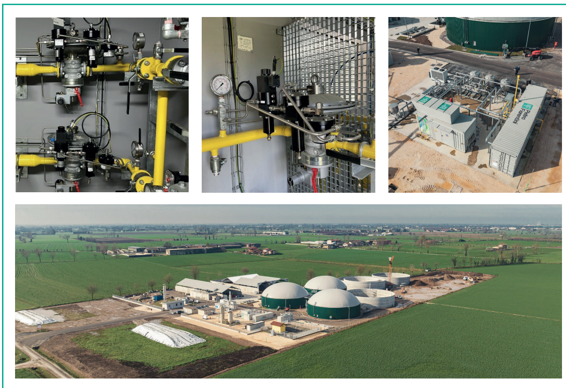
Figure 6 Biogas (RNG) upgrading and injection stations
