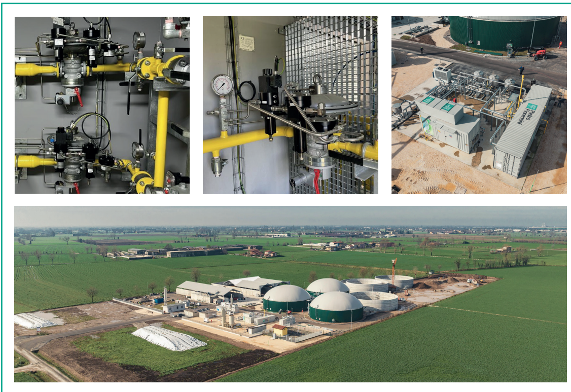
Figure 6 Biogas (RNG) upgrading and injection stations
