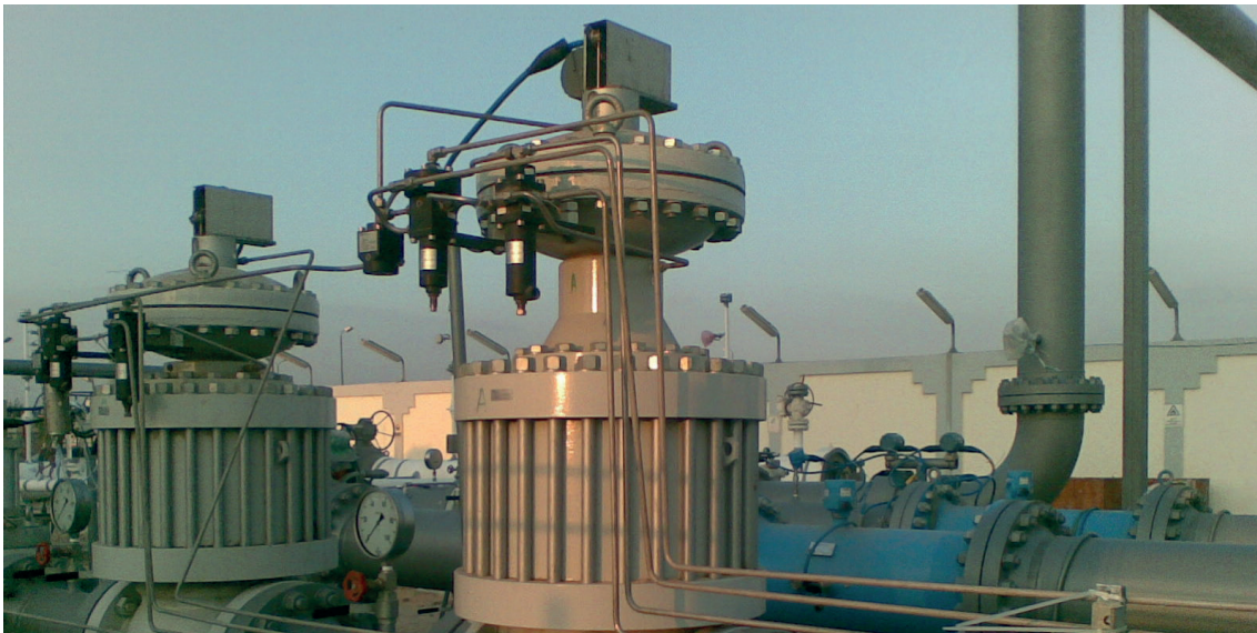
Reflux 819/FO/DB + Reflux 819/DB | Fuel gas skid per turbina a gas in EMEA
